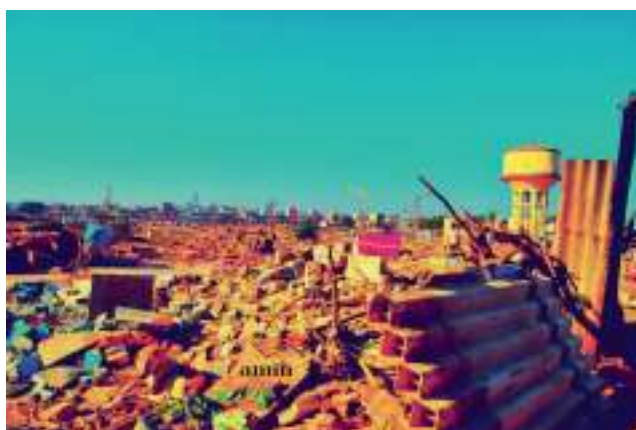
From Ejipura EWS Quarters demolition site
